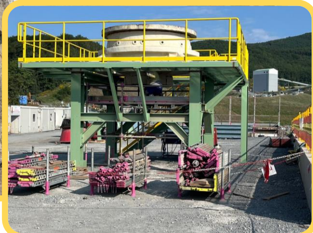
Primary crusher pre-assembly
